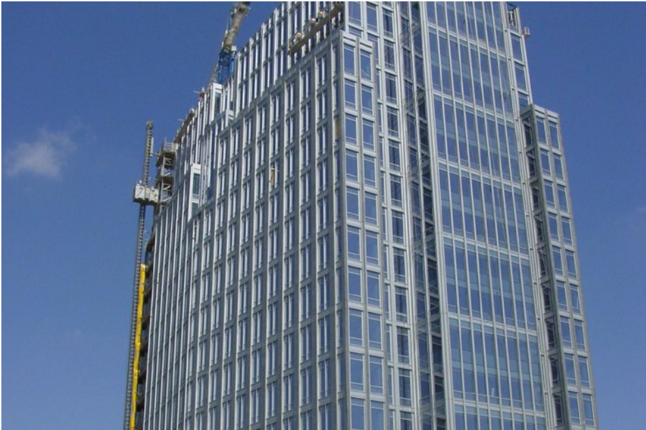
DOWSIL™ 756 SMS Building Sealant was specified on the Pier 1 Corporate Headquarters building for its compatibility with stone, metal and glass substrates as well as its ability to resist staining. [Photo courtesy of CDC, Inc.]
