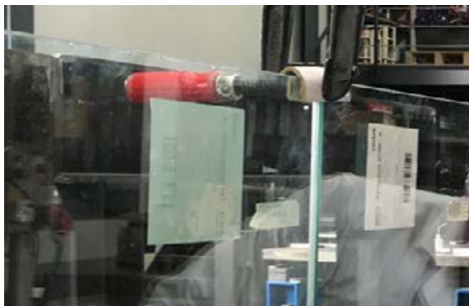
Figure 6: Connect adjacent panes using F-clamps
