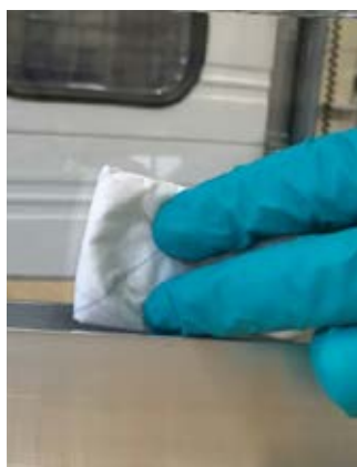
Figure 15: Cleaning the glass before applying the weather seal
