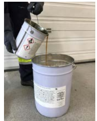
Figure 12: Pour part B hardener in part A pail
