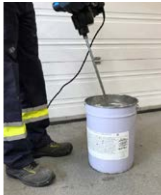
Figure 10: Mixing content of part A pail
