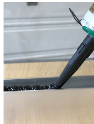
Figure 16: Applying the silicone sealant for weatherproofing
