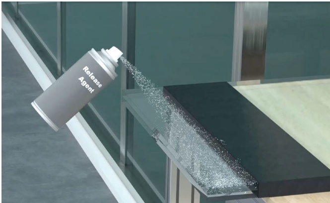
Figure 3: Spray release agent on glass
