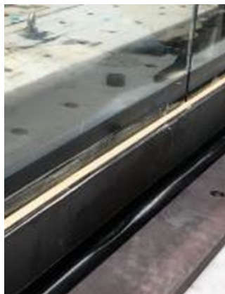
Figure 14: DOWSIL™ 375 Construction & Glass Embedding in U-profile
