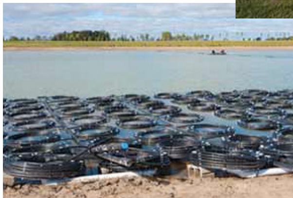
These lines are ready to be submerged and filled with DOWFROST Fluid to begin working in Saginaw Valley State University's aquathermal heating and cooling system.
