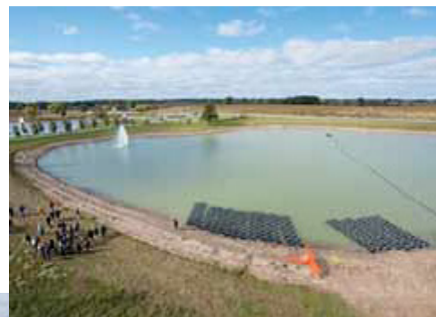
These lines are ready to be submerged and filled with DOWFROST Fluid to begin working in Saginaw Valley State University's aquathermal heating and cooling system.
