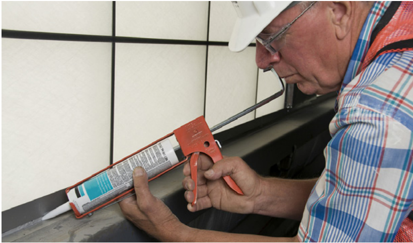
Figure 3: One component sealants (i.e. DOWSIL™ 795 Structural Glazing Sealant or DOWSIL™ 995 Silicone Structural Sealant) can be used in both factory and jobsite applications
