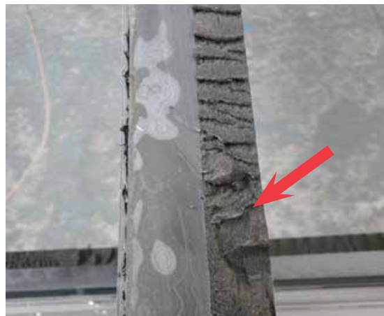
Left side photo shown incomplete joint fill (big cavity between glaze tape and sealant). Right side photo had complete joint fill (no cavity).
