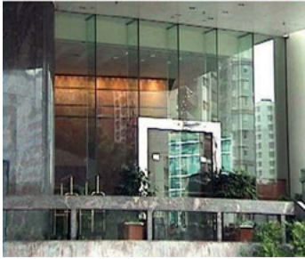
Figure 20: Typical Total Vision System at building lobby
