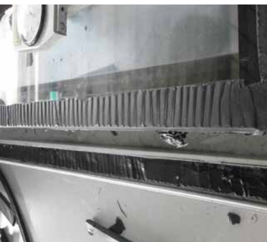
Good adhesion was found between structural sealant onto alum. frame and glass surface. Right side photo shown a large area of sealant lost adhesion onto alum frame.
