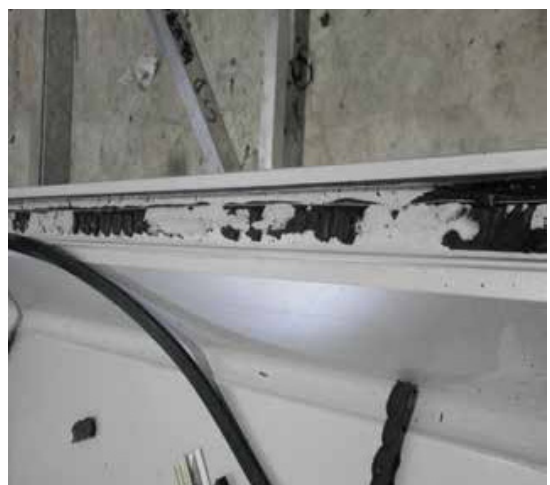
Good adhesion was found between structural sealant onto alum. frame and glass surface. Right side photo shown a large area of sealant lost adhesion onto alum frame.
