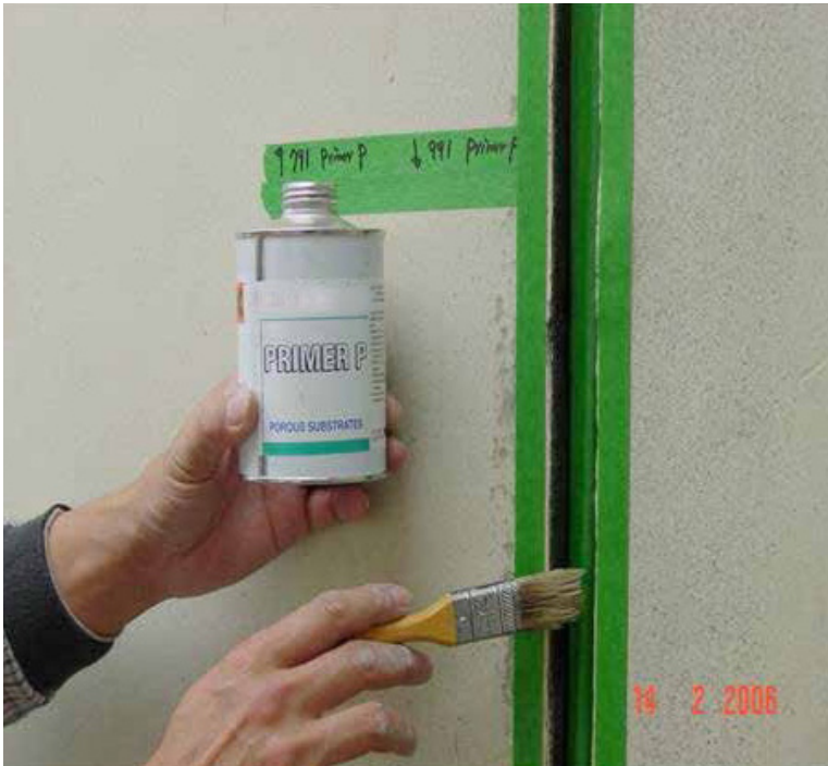
Figure 6: DOWSIL™ Construction Primer P is a film forming primer which can be applied onto concrete substrates with a brush.
