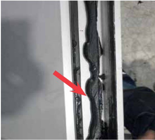
Left side photo shown incomplete joint fill (big cavity between glaze tape and sealant). Right side photo had complete joint fill (no cavity).
