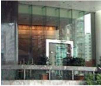
Figure 20: Typical Total Vision System at building lobby
