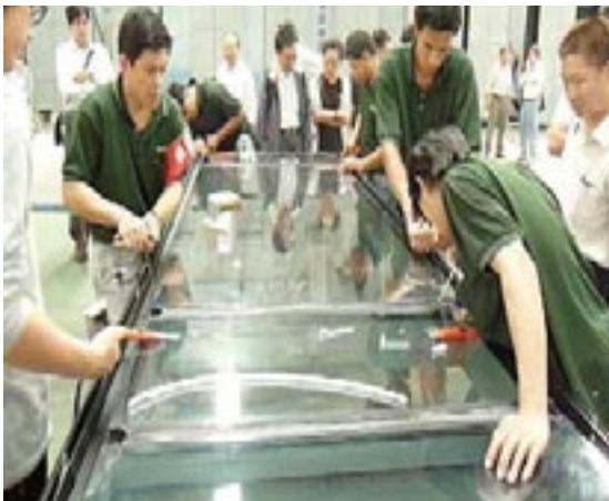
Workers using steel wire to cut open the glazed structural sealant and glaze tape (weatherseal need to remove first with knife). It can be operated at either way (both on top or one top one down)
