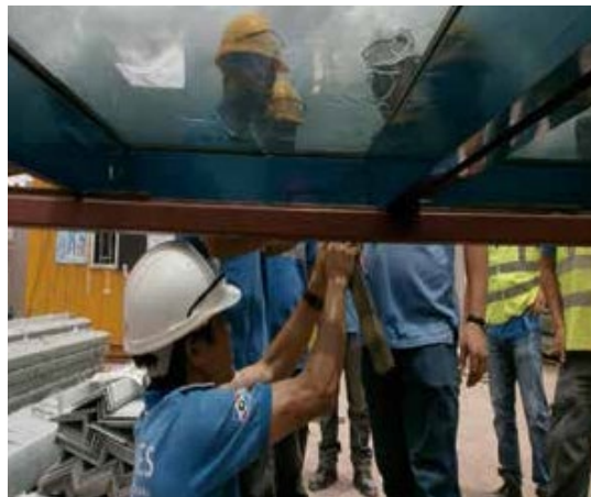
Workers using steel wire to cut open the glazed structural sealant and glaze tape (weatherseal need to remove first with knife). It can be operated at either way (both on top or one top one down)
