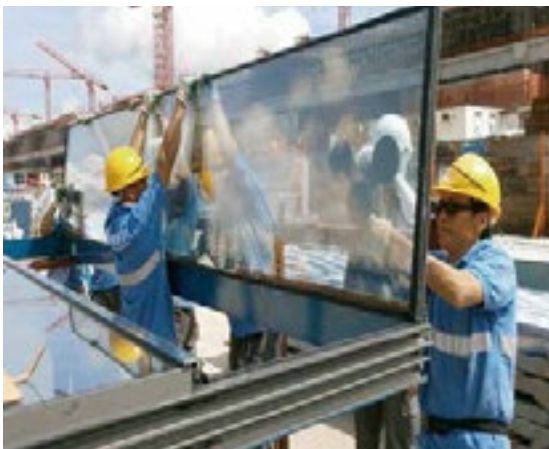
After structural joint cut open the un-glazed glass can be removed from the support frame. Right side photo shown the glass was removed then the joint fill (right photo showing excellent joint fill) and sealant mix quality can be visually check.
