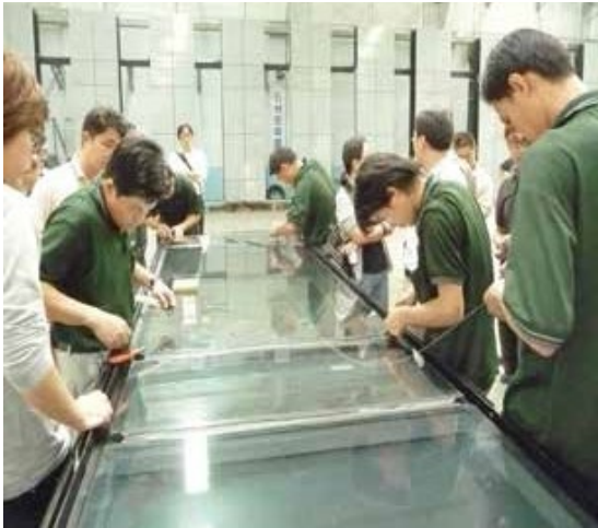
Workers put steel wire to glazed structural joint through cut open weatherseal joint (L-joint design). If structural joint can be access directly then knife or glazer can be used in cut open the sealant joint right photo).
