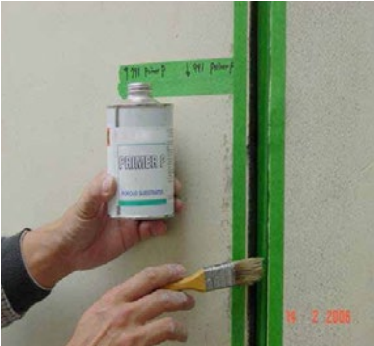
Figure 6: DOWSIL™ Construction Primer P is a film forming primer which can be applied onto concrete substrates with a brush.
