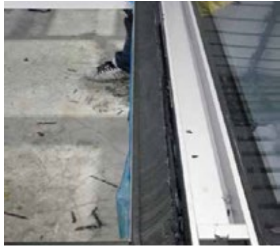
Left side photo shown incomplete joint fill (big cavity between glaze tape and sealant). Right side photo had complete joint fill (no cavity).
