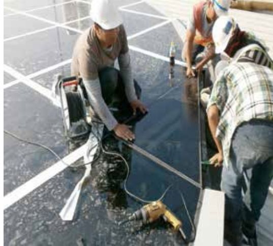
Workers put steel wire to glazed structural joint through cut open weatherseal joint (L-joint design). If structural joint can be access directly then knife or glazer can be used in cut open the sealant joint right photo).
