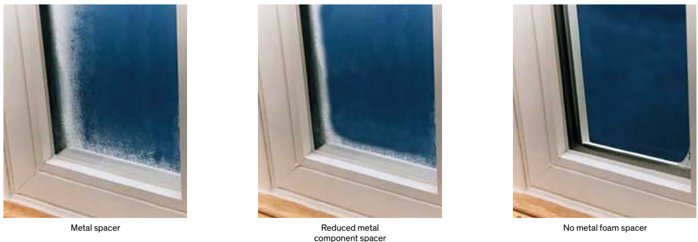
Figure 2 – Condensation and frost forming on interior pane for different spacer systems (Courtesy of Edgetech I.G. Inc., Cambridge, Ohio, U.S.A., www.edgetechig.com/ )
