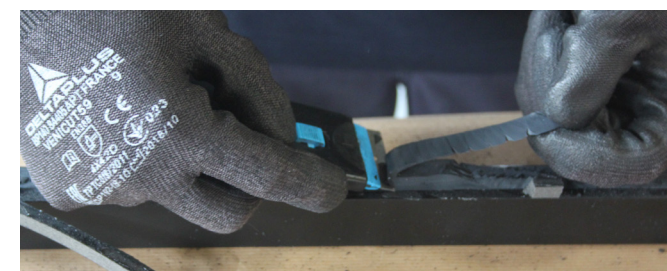
Mechanical detachment of sealant from frame
