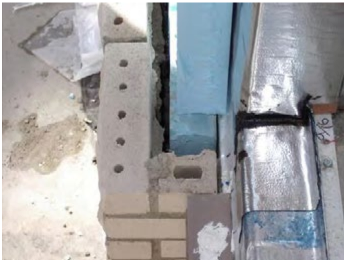
Figure 1: Self-adhered membrane installation at window opening – multiple layers and sequencing implications.
