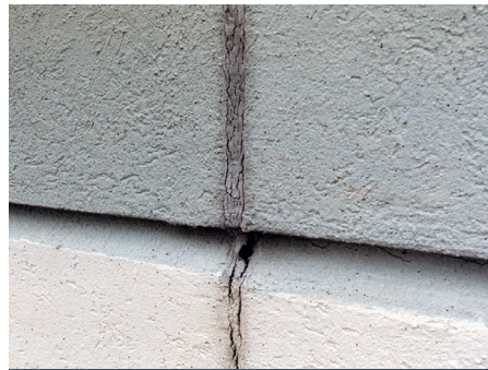
Polyurethane sealant alligating
