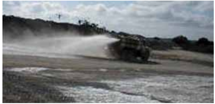
PAVECRYL™ application at loading yards.
