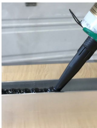
Figure 15: Applying the silicone sealant for weatherproofing
