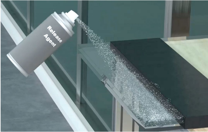
Figure 3: Spray release agent on glass
