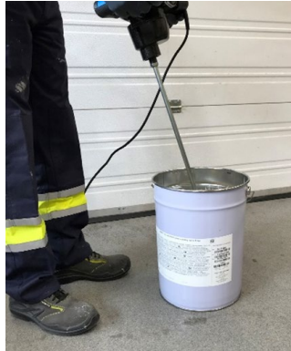
Figure 9: Mixing content of Part A pail
