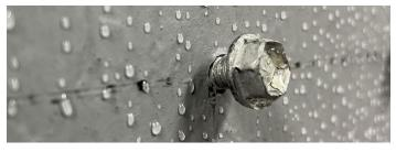
Example of a self-drilling screw fastener penetration
