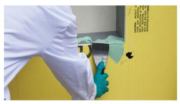
Example of using DOWSIL™ 778 Silicone Liquid Flashing
