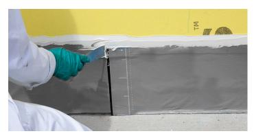
Example of bridging from below grade waterproofing to air barrier using DOWSIL™ 758 Silicone Weather Barrier Sealant
