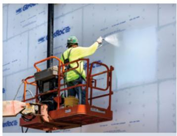
DOWSIL™ DefendAir 200 was applied to the building's GlasRoc Sheathing and concrete block substrates using an airless sprayer. Thanks to the product's excellent unprimed adhesion to most common construction materials, no primer was required.
