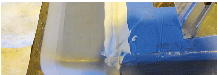
Figures 5 and 6: Strip installed with sealant under strip and over lap joint
