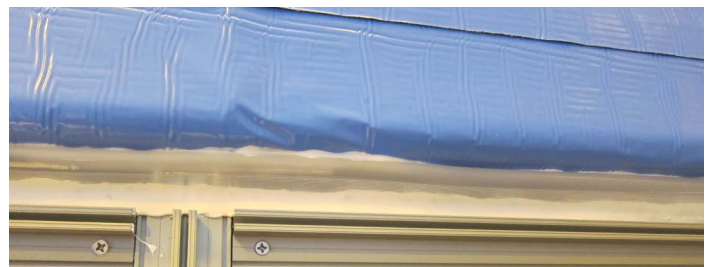
Figure 14: Finished strip installation
