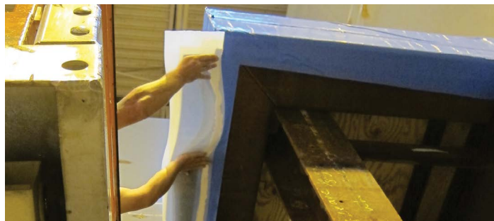
Figure 9: Installing strip at head of fenestration unit using sealant
