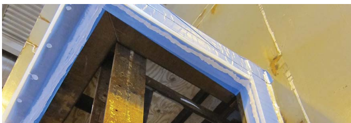
Figure 7: DOWSIL™ Silicone Transition System-wrapped opening
