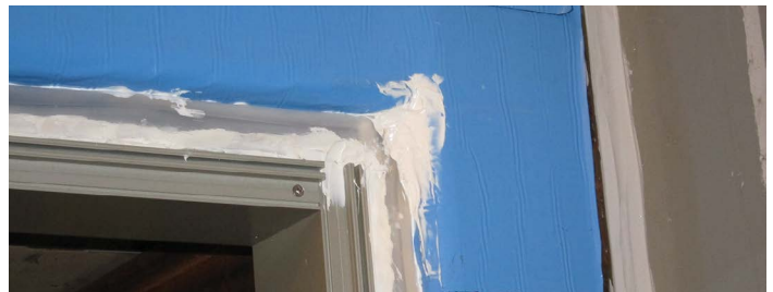
Figure 12: Folded and sealed corner
