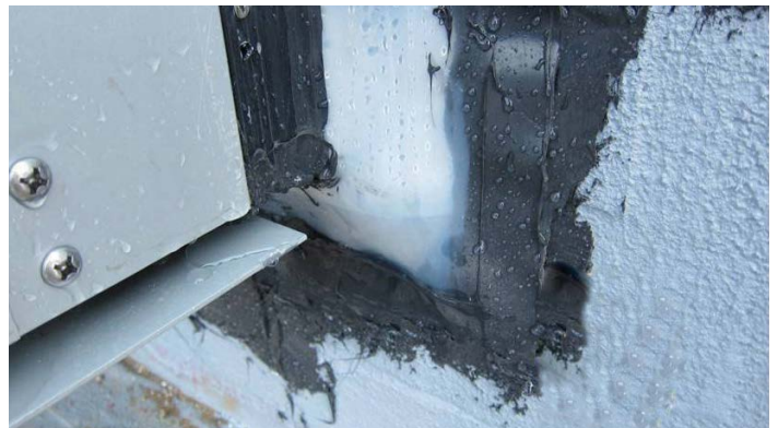
Figure 4: Sealant attaching strip and corner to air barrier in-field. Lap joints sealed.
