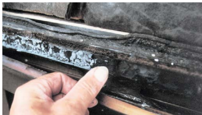
Figure 6: Residential building using silicone bonded glazing after external fire. The silicone shows a silica char.
