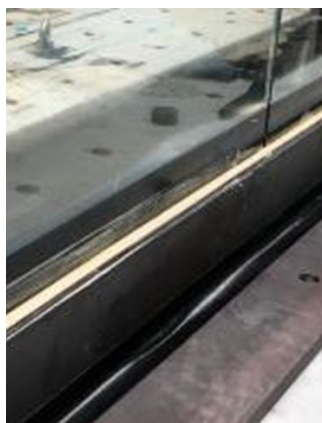
Rys. 14: DOWSIL™ 375 Construction & Glass Embedding w profilu U
