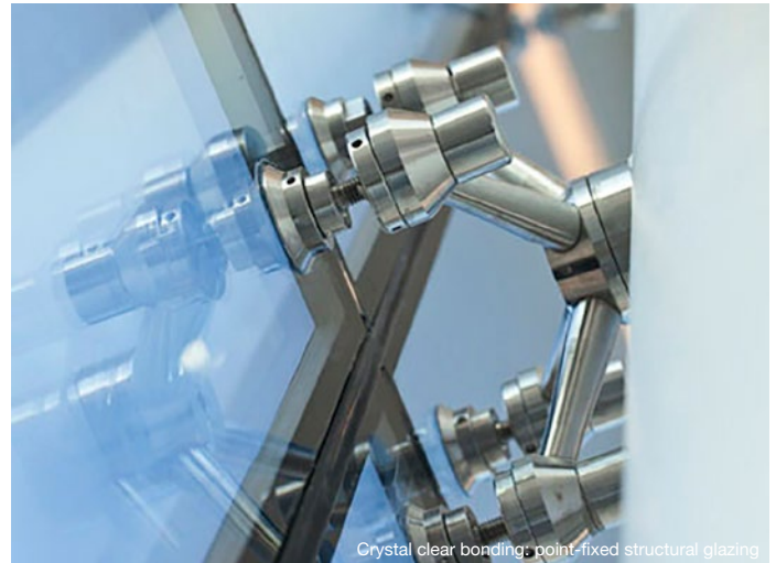
Crystal clear bonding: point-fixed structural glazing
