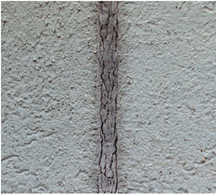
Failed urethane sealant in EIFS joint
