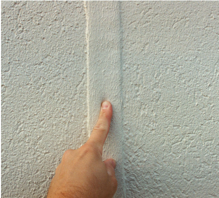
EIFS joint restored using DOWSIL™ 123 Silicone Seal
