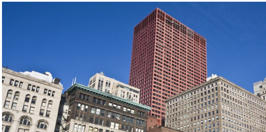
Over 2,500 window lites on the CNA Financial Plaza Building in Chicago, Illinois, were retrofitted with the 3M Ultraflex Window System, a high-performance, impact-resistant, protective window film system glazed with DOWSIL™ 995 Silicone Structural Sealant.
