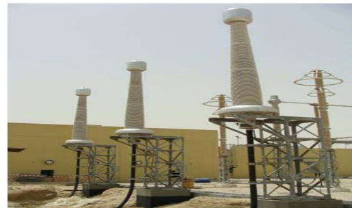
Figure 6: 400 kV Termination under construction
