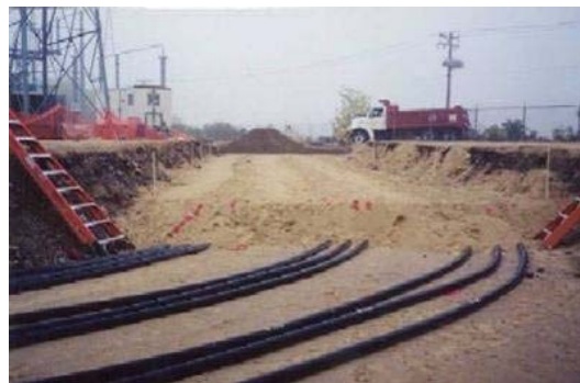
Figure 18: Installation of 400 kV XLPE cables
