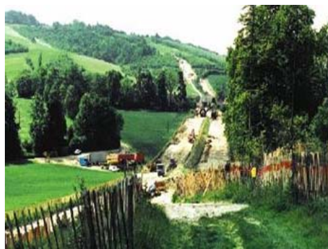
Figure 17 : cable route at site
