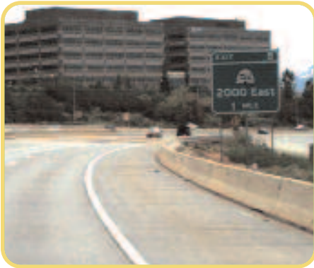
View of Utah Route I-215 in Salt Lake Valley, on PCC (Portland cement concrete) pavement. Courtesy of Utah DOT
