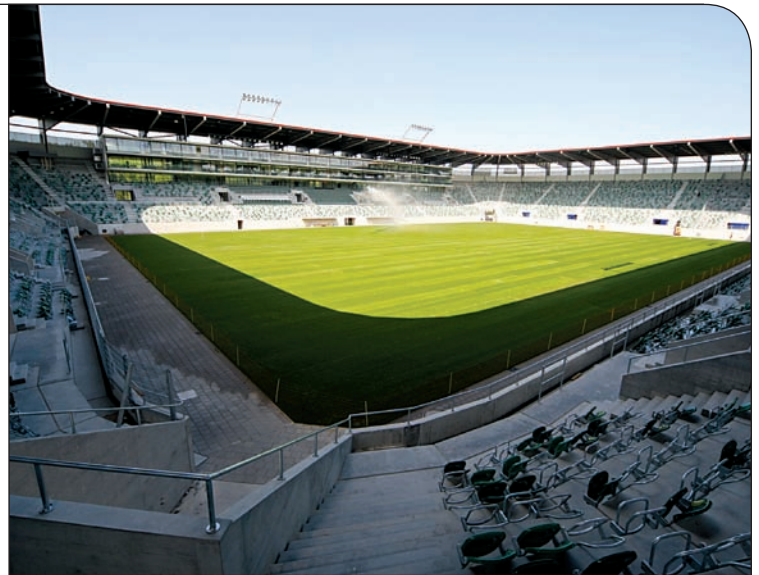
A state-of-the-art hydronic earth-warming system was built beneath the surface of the lawn to keep the field at AFG Arena in St. Gallen, Switzerland play-ready. (Photo courtesy of AFG Arena.)
